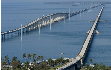
Seven Mile Bridge 1982
