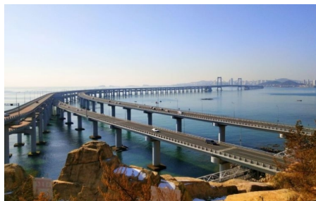
Xinghai Bay Bridge 2011
