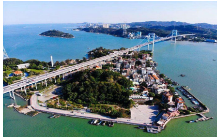
Shantou Bay Bridge 1995
