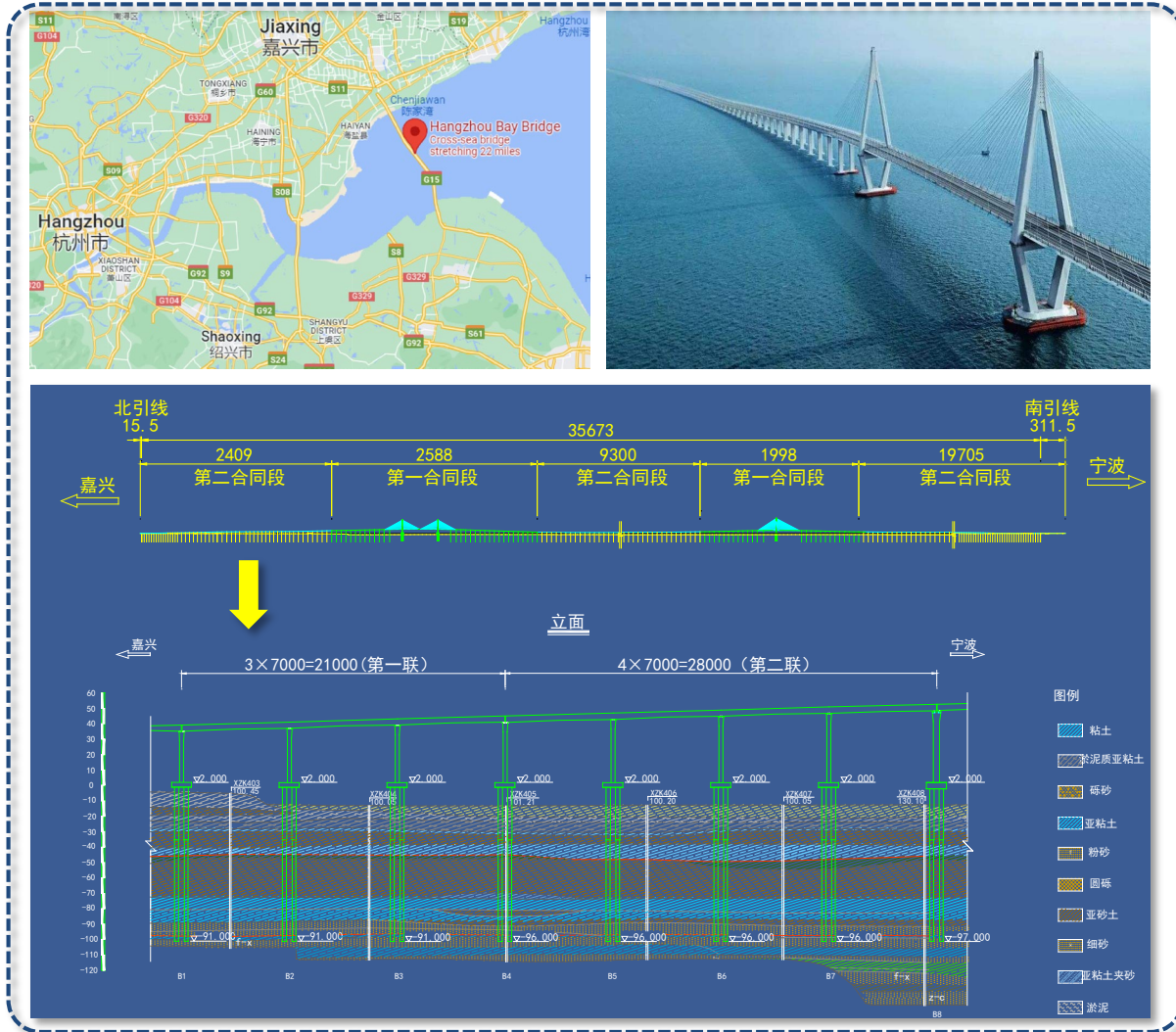
North approach bridge, Hangzhou Bay Bridge 2008
