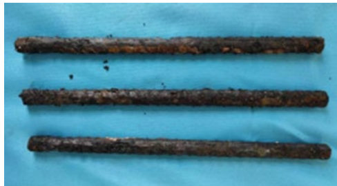
Corroded steel bars
